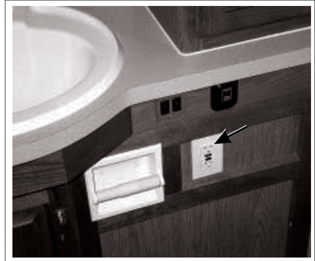
Fig. 10-4 GFCI OUTLET (TYPICAL)
